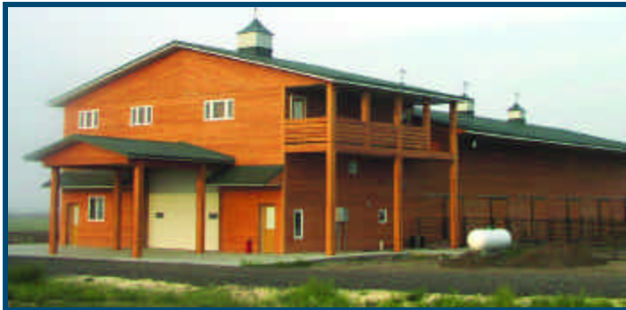
Reward ICFs made this unique house/barn combination at Proven Sires Ranch practical and easy to build.
