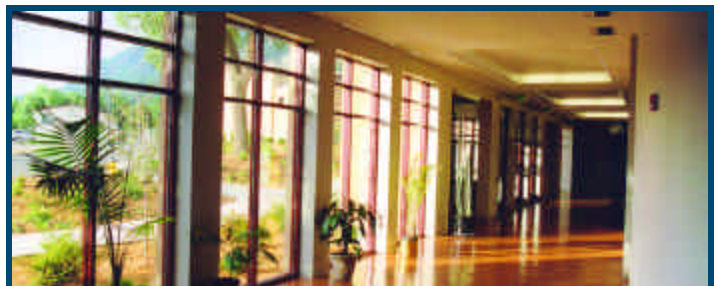
Both the exterior and the interior bearing walls were built using Reward ICFs
