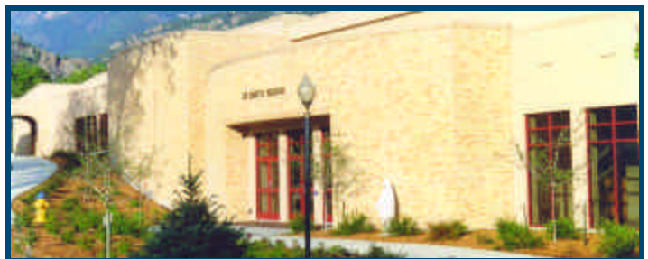
The archway (left) shows where the wedge-shaped addition connects to the school. The doors lead into the 400-seat auditorium.
