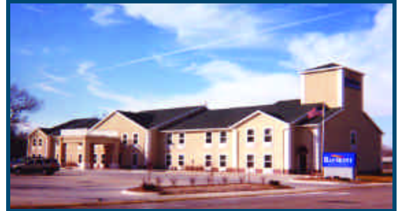
The Baymont Inn & Suites in Salina, Kansas, is typical of the types of commercial projects Reward ICF professionals all over the country are building.
