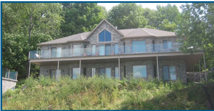
Energy efficient Reward walls allow the owners of this house to get by without air conditioning.
