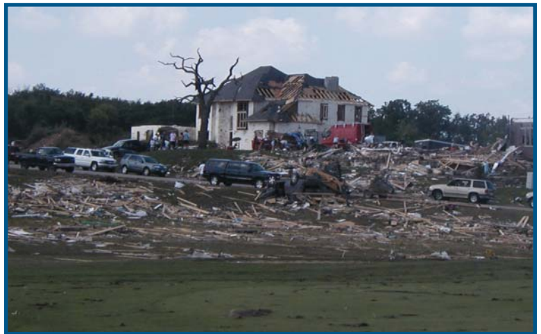
Reward stands alone. This house, built with iForm, withstood the F-3 tornado that destroyed neighboring homes.
