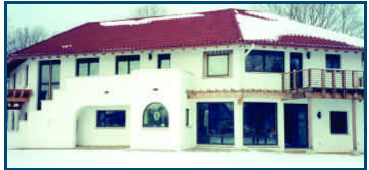
Curved windows were easily accomplished with Reward forms
