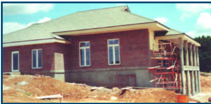
Built for durability, the meeting house features concrete floors, columns and deck in addition to the ICF walls.
