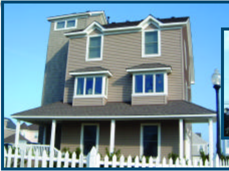
This all-concrete beach house was built to last. Inset: Vandergrift accomplished the all-concrete decks and column by building in lifts.
