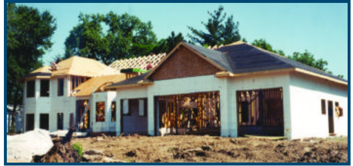
Work progressed quickly despite a high wind setback.
